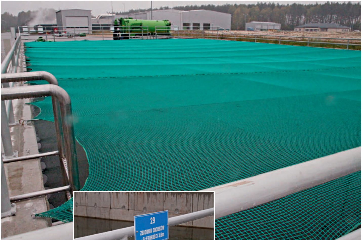
Process water store ▲ Prozesswasserspeicher
